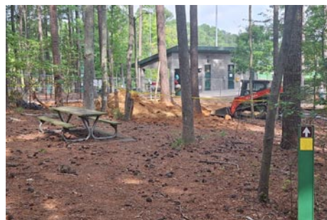
Sidewalk construction stalls at Cedar Falls. PHOTO BY SUSAN KELLY
